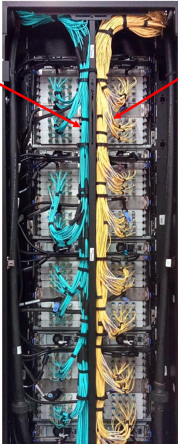
Figure 38: Fiber Optic Cables in Spine (Structured Breakout Cables on Left, Point-to-Point Cables on Right)
