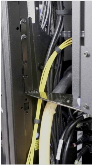
Figure 49: Example, Fiber Optic Cable Routing
