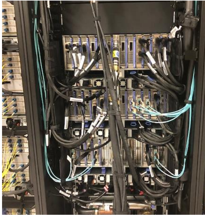
Figure 52: CPC Short Range Coupling Cables Routed to sides of frame
